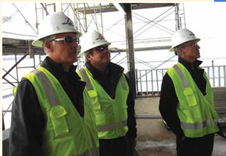
Aspen Valley Hospital board president John Sarpa, board member Lee Schumacher, and board treasurer Chuck Frias tour the construction site.
