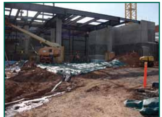
The underground parking structure is now easily identified.
